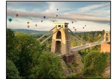
Clifton Suspension Bridge
