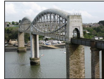
Royal Albert Bridge
